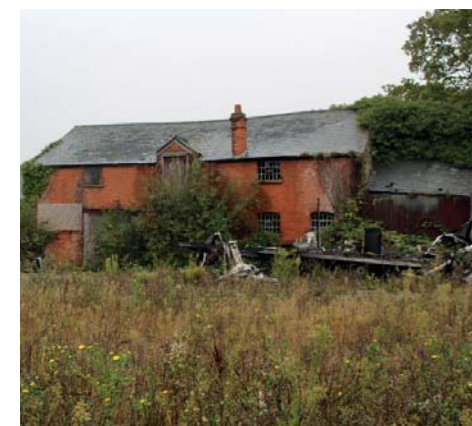
Figure 16 The stables and coach house of the King Edward Public House
