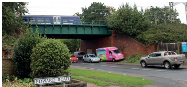
Figure 21 Thorpe-le-Soken railway bridge
