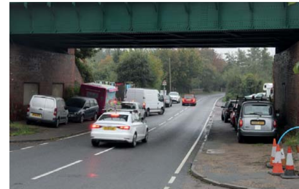
Figure 53 Cars parked under the rail bridge on the edge of the Conservation Area
