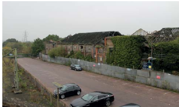
Figure 39 Viewpoint 2 looking north-west
